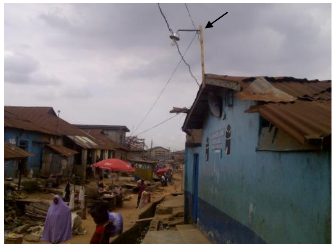
One of the street lights locally made by the VPS groups
